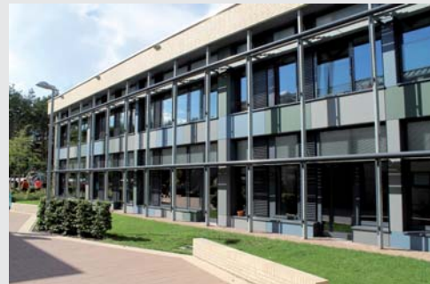
Energy surplus school at Hohen Neuendorf
