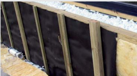
Mounting the facade insulation at Hedegaards School
