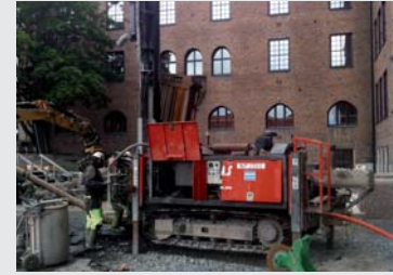
Heat pump, geothermal drilling
